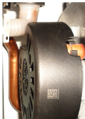
Flow of condensate on the fan.
